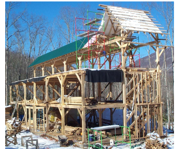
A timberframe condo built with lumber sawn from a small sawmill
